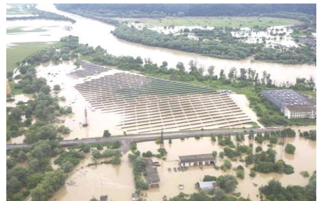
A flooded solar power plant
