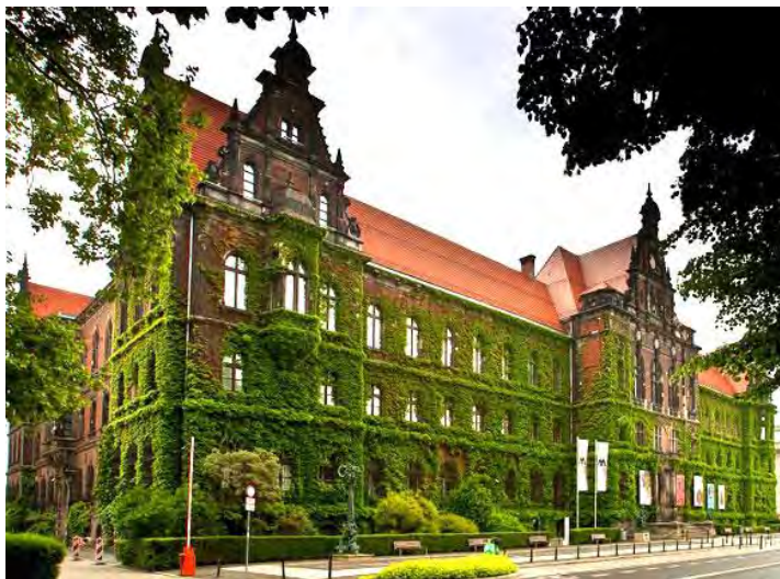
Fig. 5. Green facade on the building of the National Museum in Wroclaw [19]
